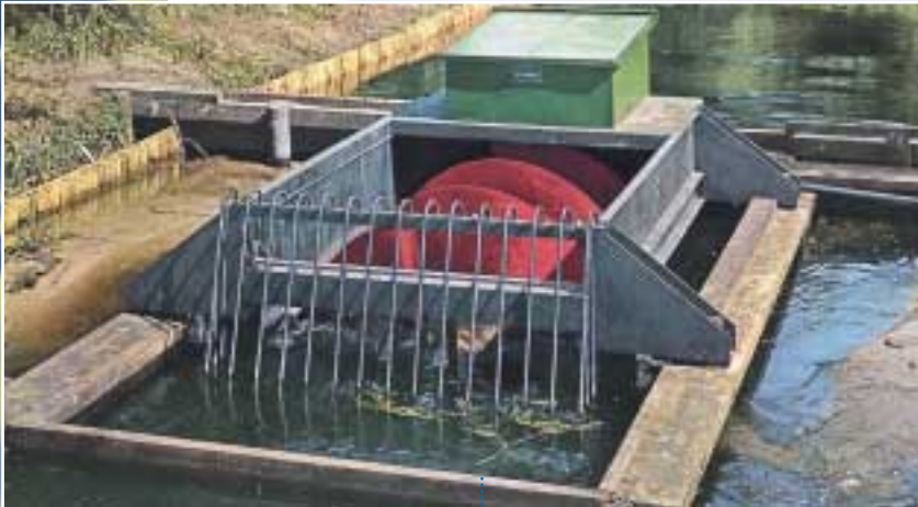
Horizontal Flushing Installation
