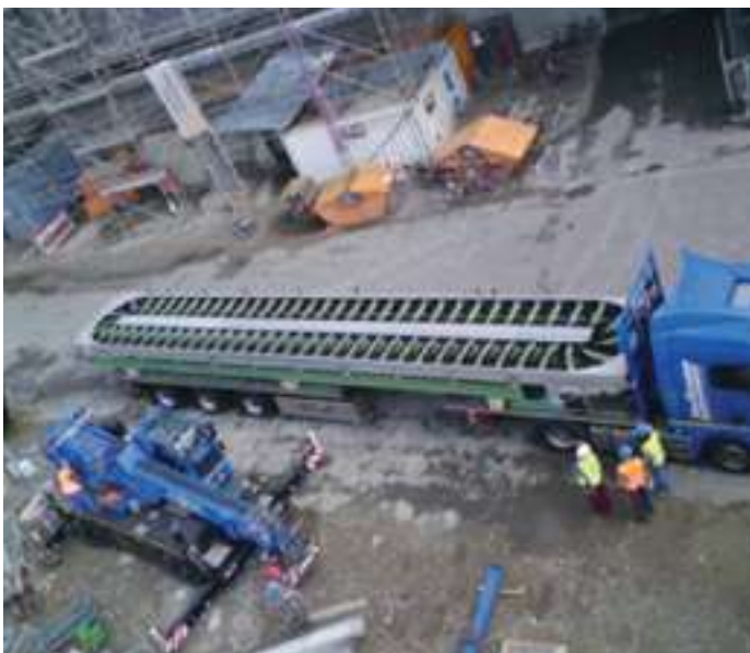
GKM 9 Power Plant, Mannheim, Germany
