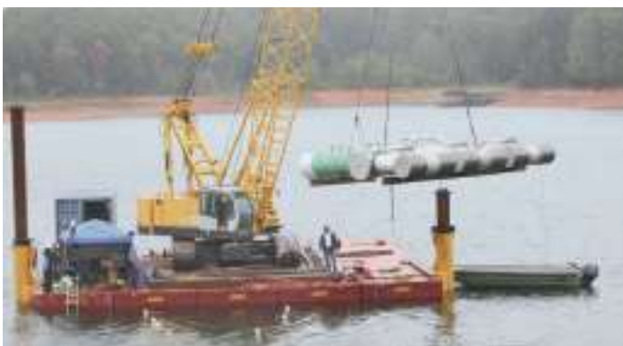
Johnson Offshore Intake Systems™ (JOIS™) Installation
