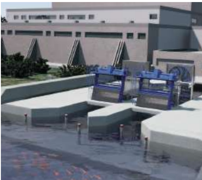
Two Channel Water Intake with Geiger® Fish Repelling and Geiger® Fish Return System
