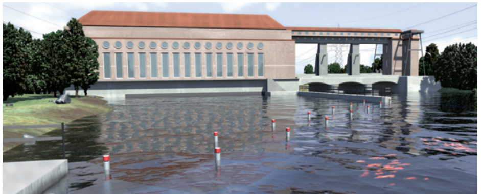
River Power Plant with Electric Fish Repelling System
